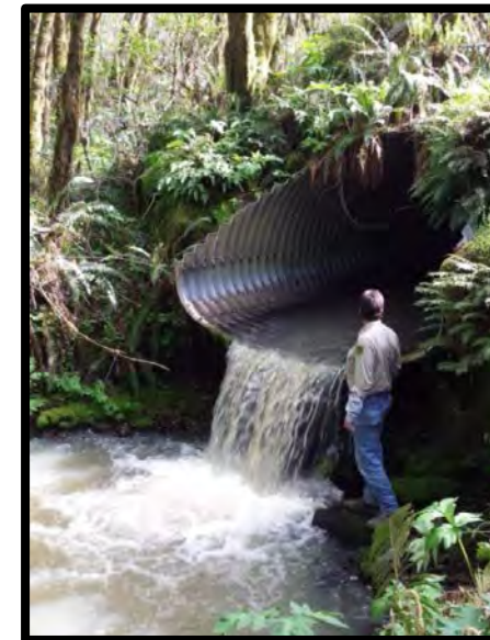
Observed potential fish passage barrier on Russell Creek, a major tributary to Dement Creek
