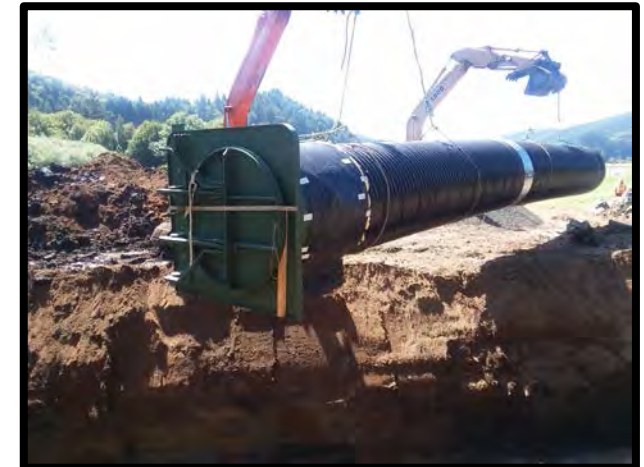
New tidegate structure installation in late July 2017
