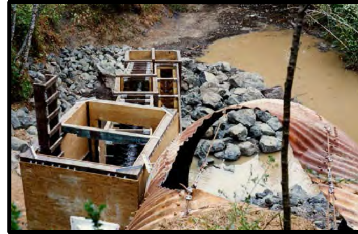
Current fish ladder that provides poor fish passage and is in need of maintenance
