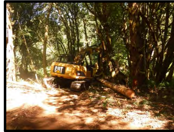
Excavator placement of LWD at one of the installation sites on Woodward Creek
