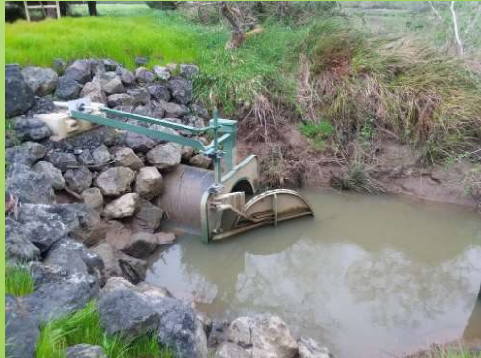
Newly replaced fish-friendly tidegate: 6'x60' Trench Coat culvert with Nehalem Marine Tidegate
