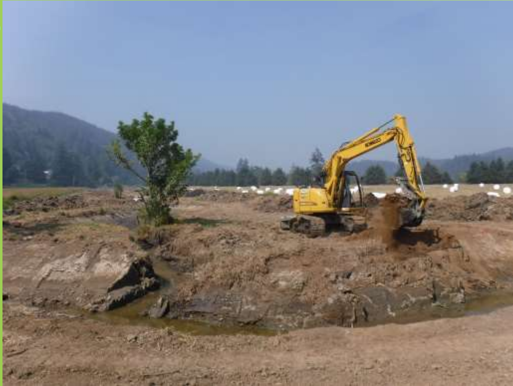
Beginning pond excavation at intersection of east/west and north/south tidal channels
