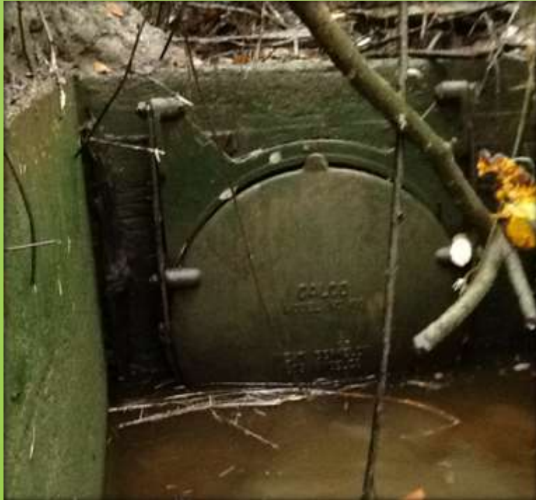
Inadequate tidegate before replacement
