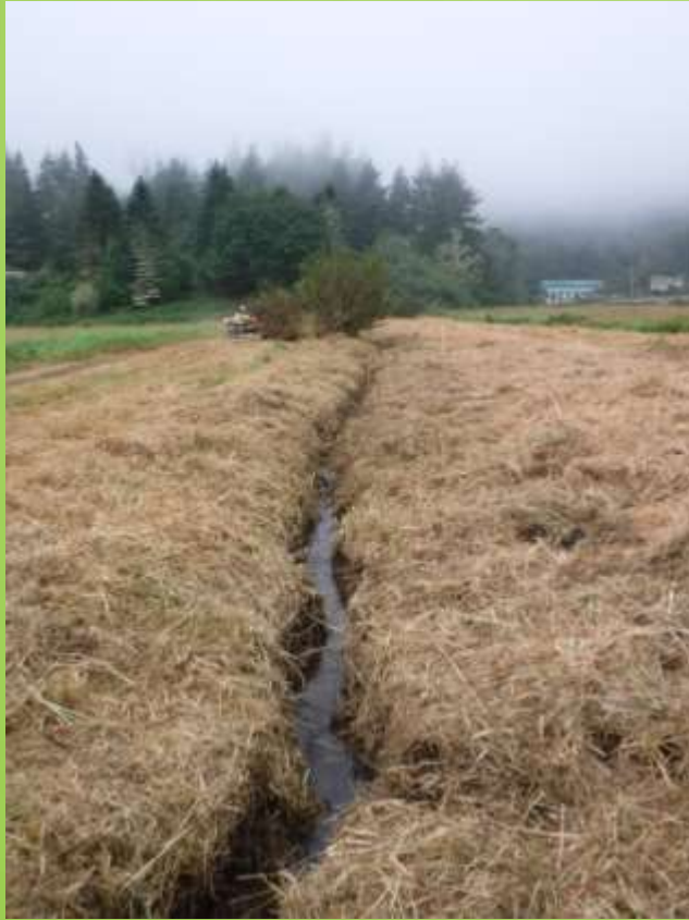
Existing tidal channel after mowing by Wheeler Excavation
