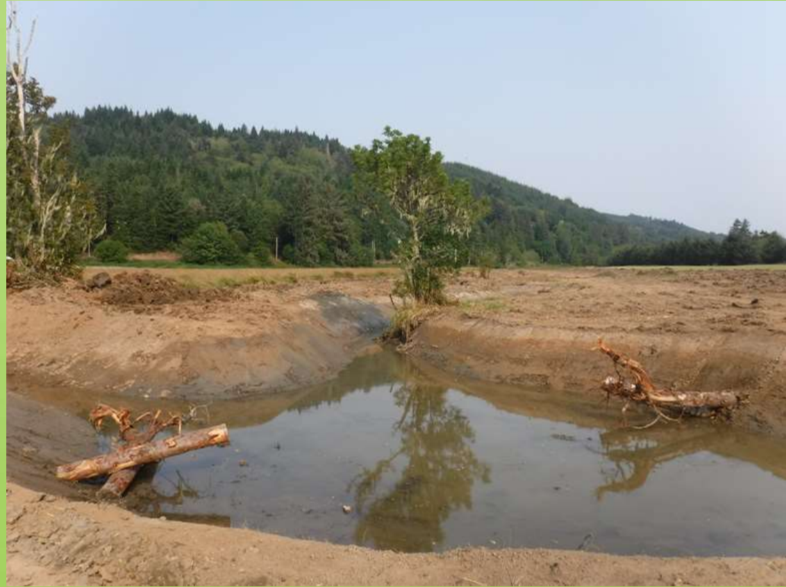
After channel construction
