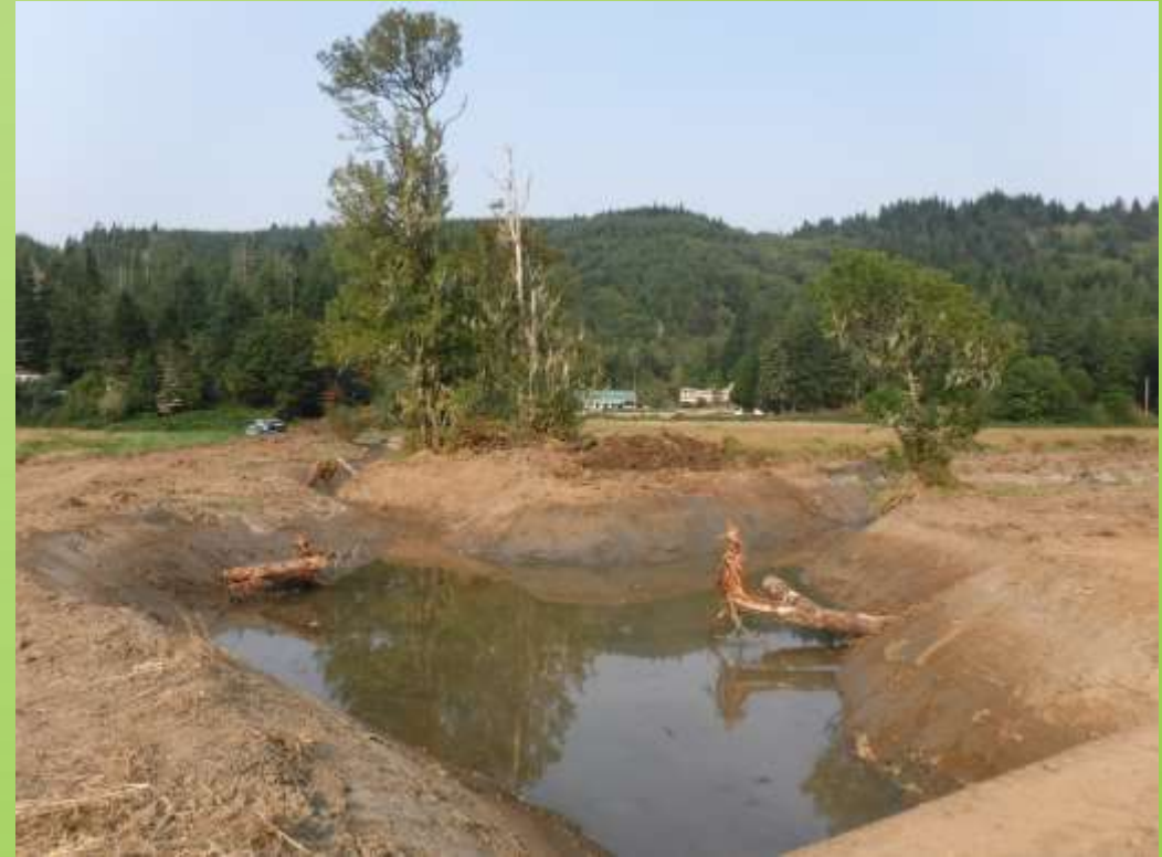
Completed pond excavation with select LWD installed
