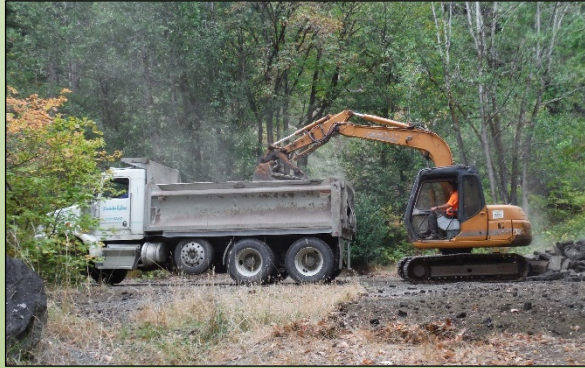
A & R Construction did a stellar job on the debris removal
