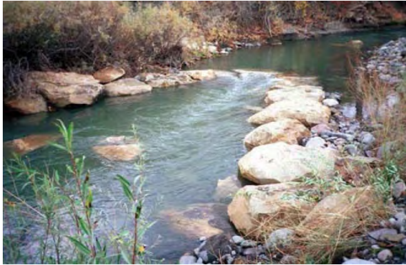
Figure 49: Cross vane on the Rio Blanco, CO (NRCS 2007, Ch11).
