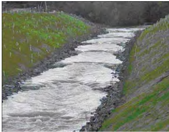
Figure 32: Pool and weir fishway.
