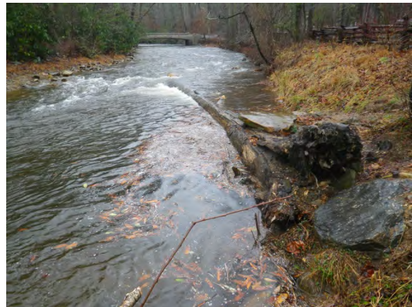
Figure 40: Log J-hook vane providing bank stabilization and pool scour 4 years after construction (Pisgah National Forest, North Carolina; photo credit: Brady Dodd).
