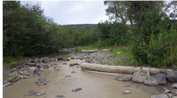
Figure 39: Log vanes providing bank stabilization and channel narrowing 2 years after construction (Milk Creek, Colorado).
