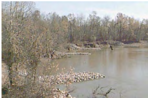
Figure 41: Bendway weir (Lagasse et al. 2009)
