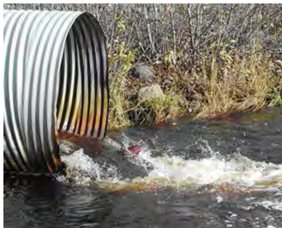
Figure 31: Culvert outlet drop, with Coho.
