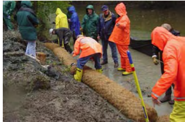
Figure 43: Installation of coir fascines (NRCS 2007, TS14I).
