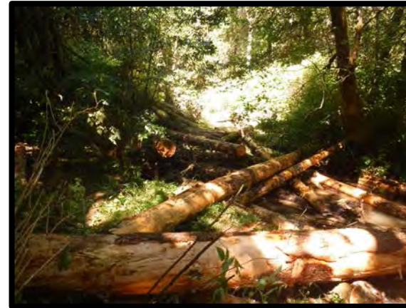
Completed LWD structure on Woodward Creek in summer of 2016
