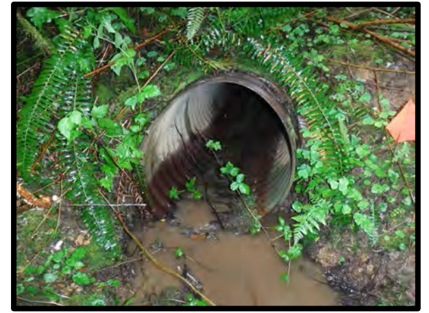
One of the culverts that will be removed during the road decommissioning.
