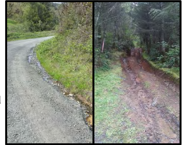
Example of sediment runoff from the road network in the basin.
