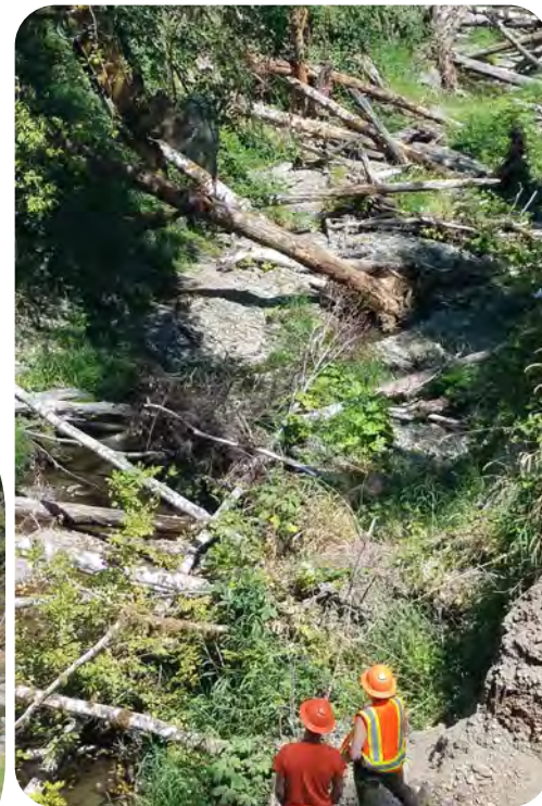
Large Woody Debris Installation, Summer 2020
