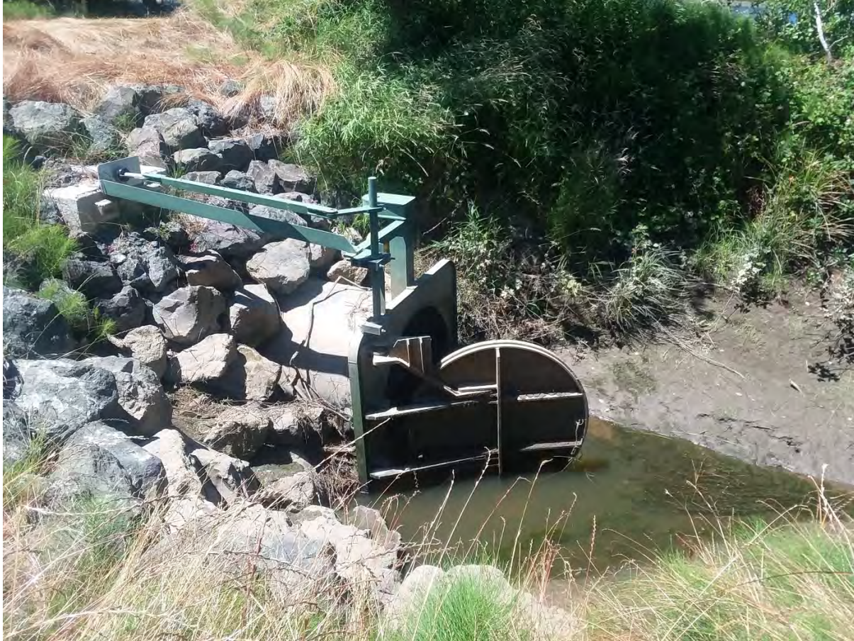
Figure 2. A 6' diameter aluminum side-hinged MTR tide gate was installed at the Cochran project in 2017. The tide gate door is installed on the riverside of the culvert.
