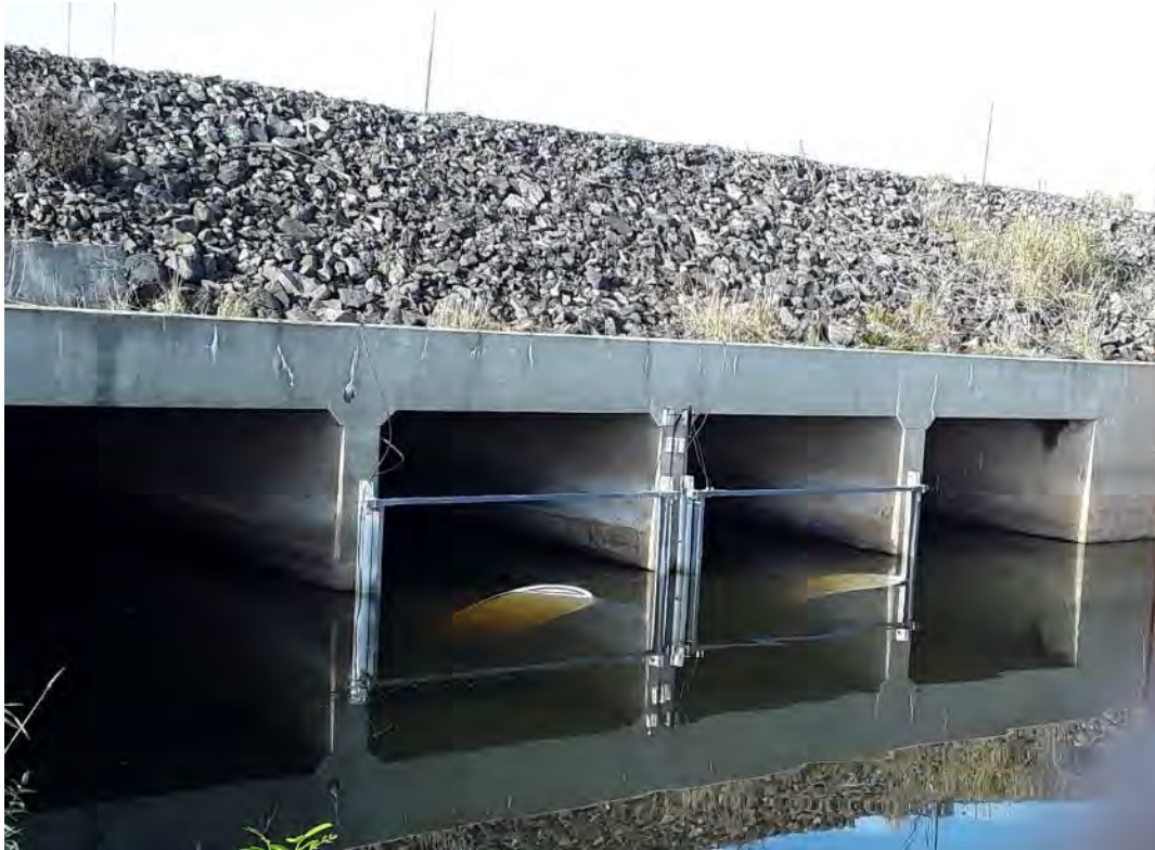
Figure 6. Winter Lake Unit 2 PIT antenna array on tide gate culvert 2B and 2C. The pass thru (gray fiberglass structure) and sail (white sail in water) antenna are installed on the landward (upstream) side of the tide gate culvert whereas the tide gate doors are installed on the river (downstream) side of the tide gate culvert.
