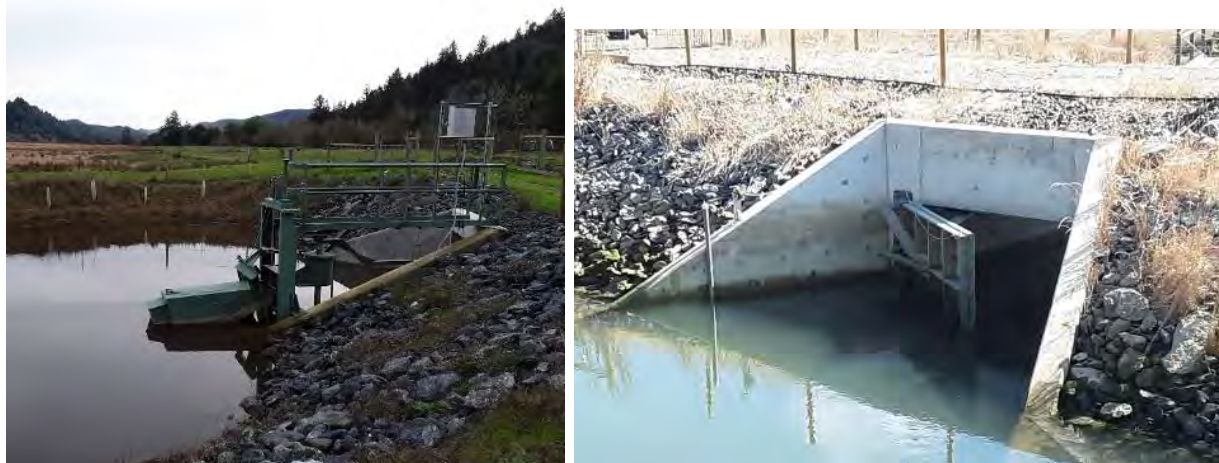
Figure 5. An 8'x8' aluminum side-hinged MTR tide gate was installed at the Seestrom project in 2019. The landward side of the MTR structure uses a counter weight to keep the tide gate door open during rising tides (left photo). The tide gate door is installed on the riverside of the concrete culvert (photo right).
