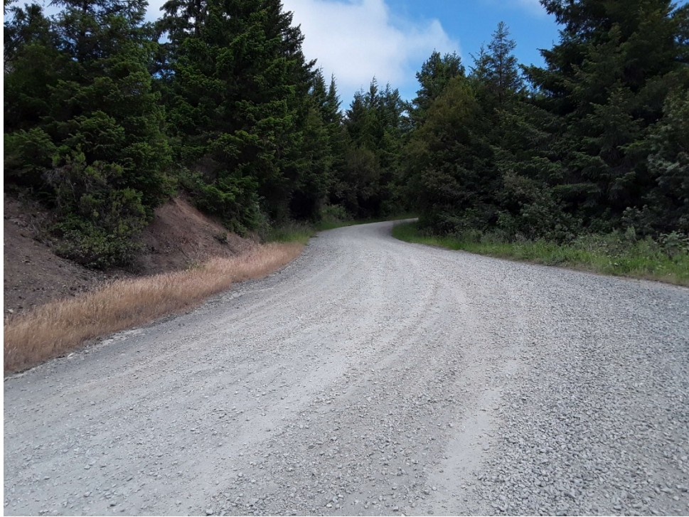
Figure 3: Eckley Mountain Road. Notice it's a steep, rocky road with no drainage culverts. Rainfall will quickly wash this road out and deposit the sediment into the creek.
